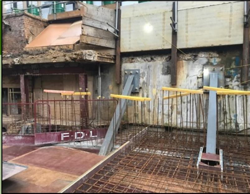
Extensive temporary works were encompassed within the demolition of Ergon House and 9 Millbank. For Ergon, the building was propped over 3 floors using over 950 heavy duty floor props and in 9 Millbank adjustable kwikform props were used as floor and internal walls were removed. Custom raking props were also installed to support the basement retaining wall following demolition of Ergon House. All propping schemes were designed in house and installed by our competent demolition team.
