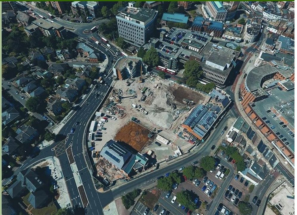
As Principal Contractor, Wooldridge Demolition carried out the demolition works of three reinforced concrete framed office blocks; Argyll House, Frances House and Brook House using two high reach machines for the majority of the works. The demolition of one of the blocks in particular required careful evaluation from the management team due to the complexity of the original structure.
